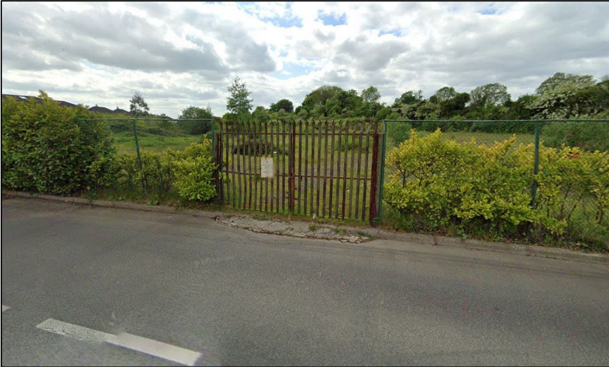
Figure 5.1: Site access point (Source: Google Maps).
